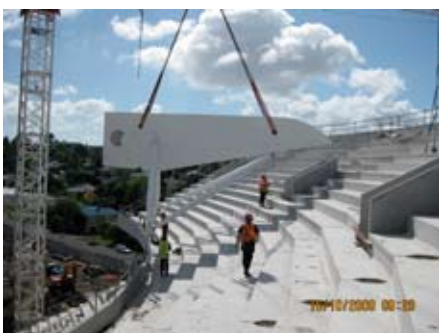
REAR GIRDER BEING LIFTED INTO PLACE.
