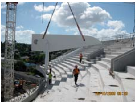
REAR GIRDER BEING LIFTED INTO PLACE.
