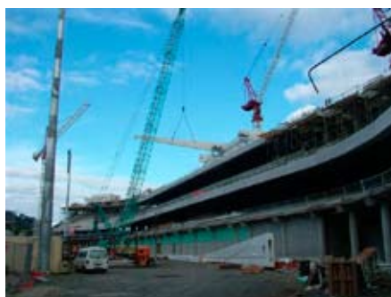
MID GIRDER SECTION BEING LIFTED INTO PLACE.
