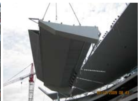
FRONT GIRDER AND INFILL SECTION BEING LIFTED INTO PLACE.
