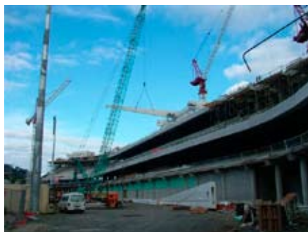
MID GIRDER SECTION BEING LIFTED INTO PLACE.
