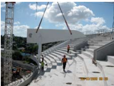
REAR GIRDER BEING LIFTED INTO PLACE.
